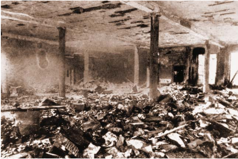
This is a photograph of the gutted tenth floor of the Asch Building that was taken in the aftermath of the fire.
